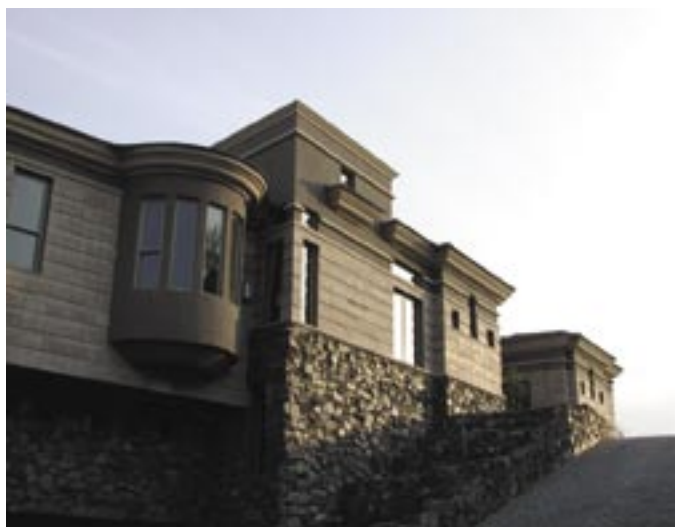
North elevation clad with stone excavated from site and cut ancient stone above
